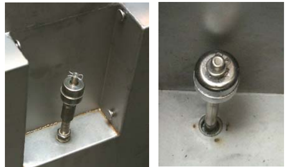
Figure 1: The float switches (above and right) should be cleaned periodically to eliminate starch buildup, which can impede the motion of the floats. Care must be taken, however, to ensure the shafts are not dislocated or the movement of the float hindered.
